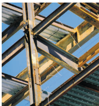
Figure 1-4 As a result of chemical change, bright steel girders become rusty when exposed to moist air.
